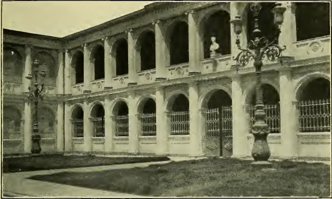
A. FAÇADE OF THE ENGINEERING SCHOOL, UNIVERSITY OF CARACAS, VENEZUELA.
